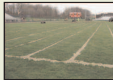
May 2007. Grand Blanc High School athletic field after the drain line installation process, Grand Blanc, Mich., Water Management Inc.,
